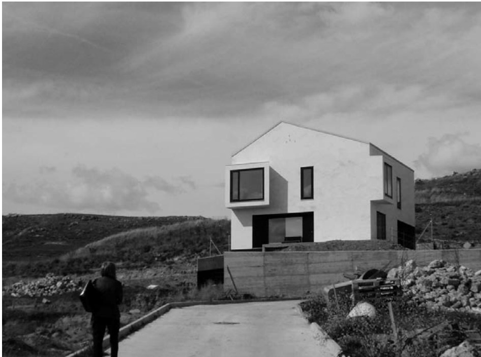
Fig. 2. TP House, Albillos, Burgos, under construction
