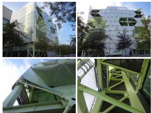
► Fig. 4: Barcelona Growth Centre in Barcelona (Spain), previously named MediaTIC. Case study in Post-Occupational Behaviour Research in Adaptive Facades.
