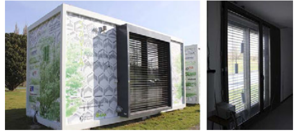
► Fig. 1: P4 Prototype. Sunspace with vertical solar heat storage. Images of University Campus in Pamplona (Spain).
