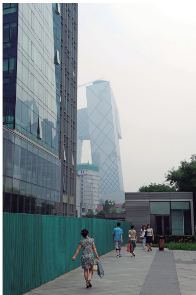
f5_One of the many different ways the CCTV building presents itself in the city Beijing, 2012
