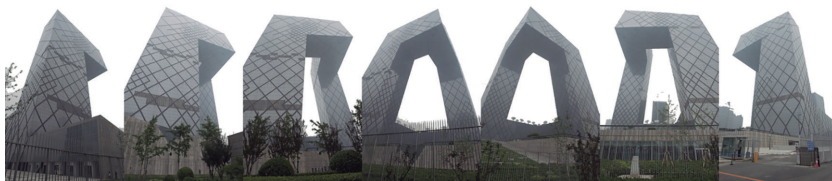
f6_Collage of the constant changing experience of representation of the CCTV building in its context Beijing/Umeå, 2012, Katja Hogenboom
