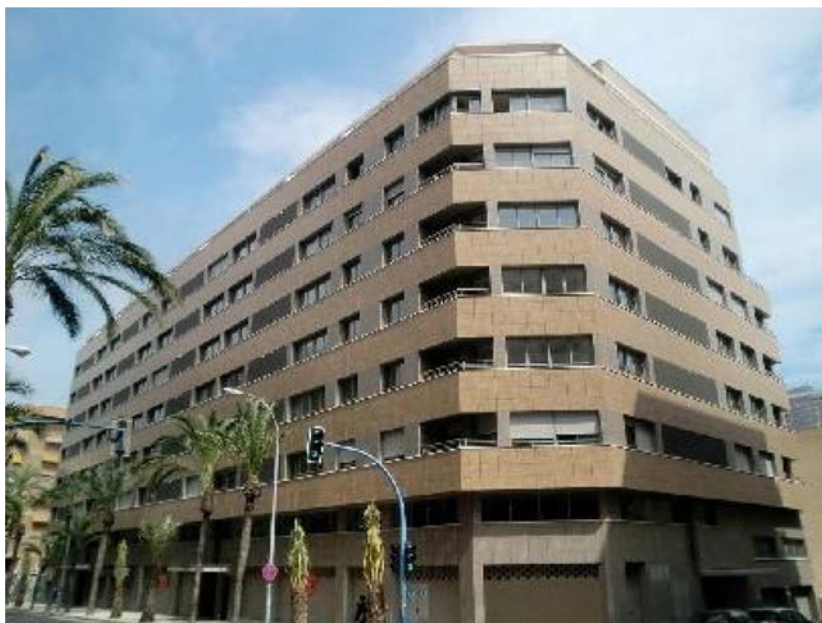
Figure 1: Typical view of the residential building. Current state.
