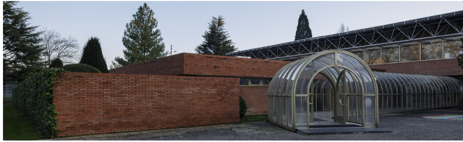
Fig. 3. Office building, School of Architecture (University of Navarra) [35].
