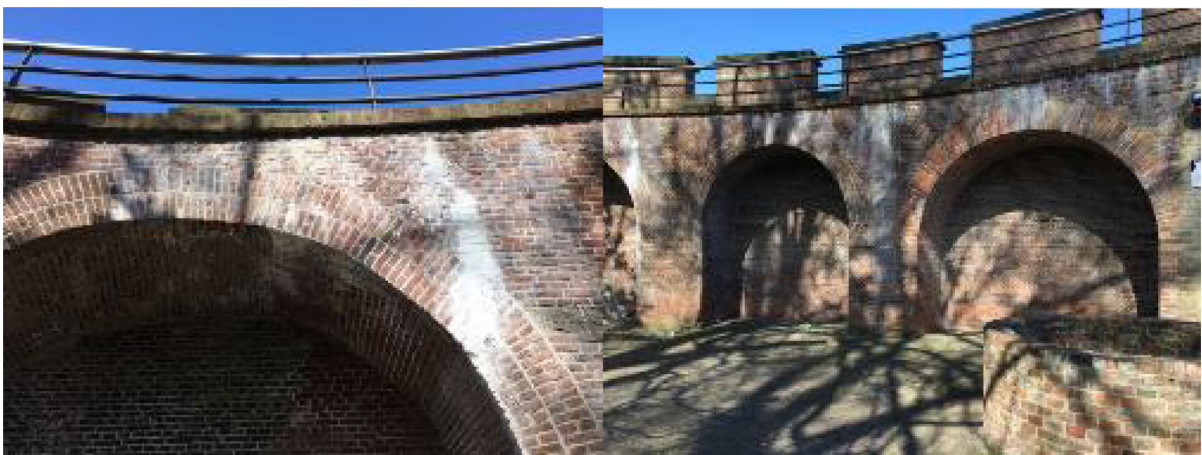
Fig. 16 Lime leaching after repair of historic masonry; see also 4.7
