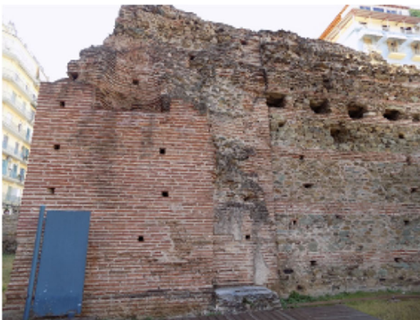
Fig. 13 Repaired masonries of Galerius Palace, as they are now
