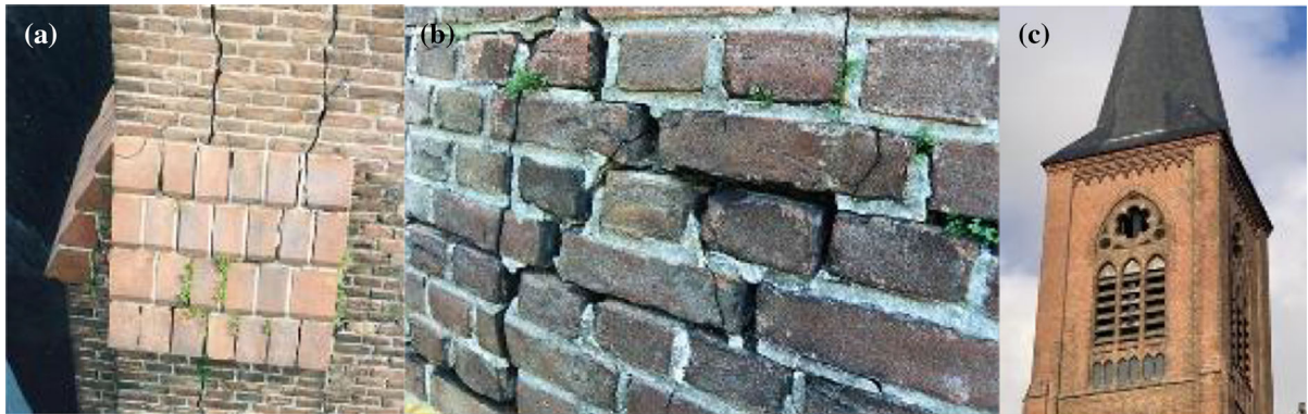
Fig. 19 Cracks in masonry, caused by expansion of bedding mortar, deeper in the wall section, due to formation of thaumasite (a); push out of the pointing is a secondary effect (b); situation several years after repair: no recurrence (c)
