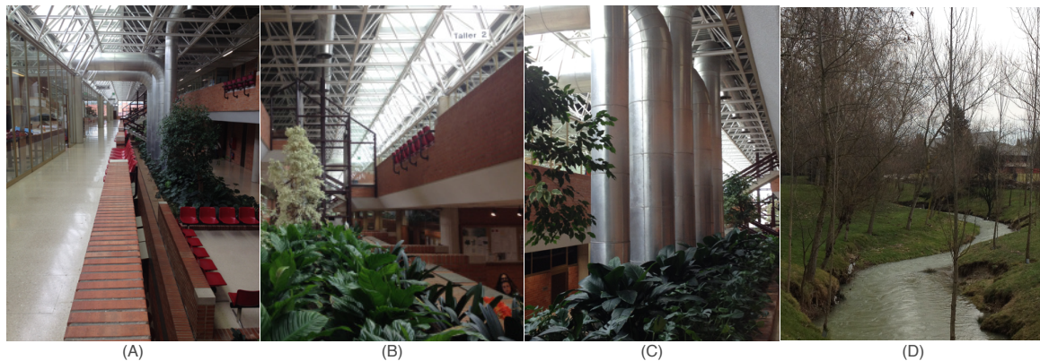
Figure 5. (A,B) Skylight in the central area of the building and the brick configuration of the walls. (C) Ducts for air distribution. (D) The Sadar River.
