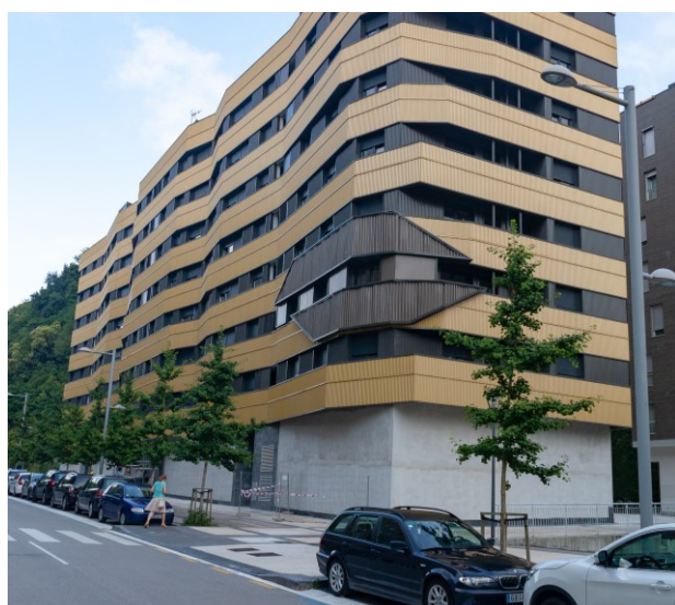
Fig. 1. Demonstration building, with the bio-based external envelope enclosing a corner apartment on the second floor.
